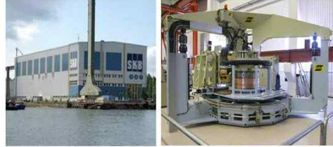
Canister laboratory, in operation since 1998
